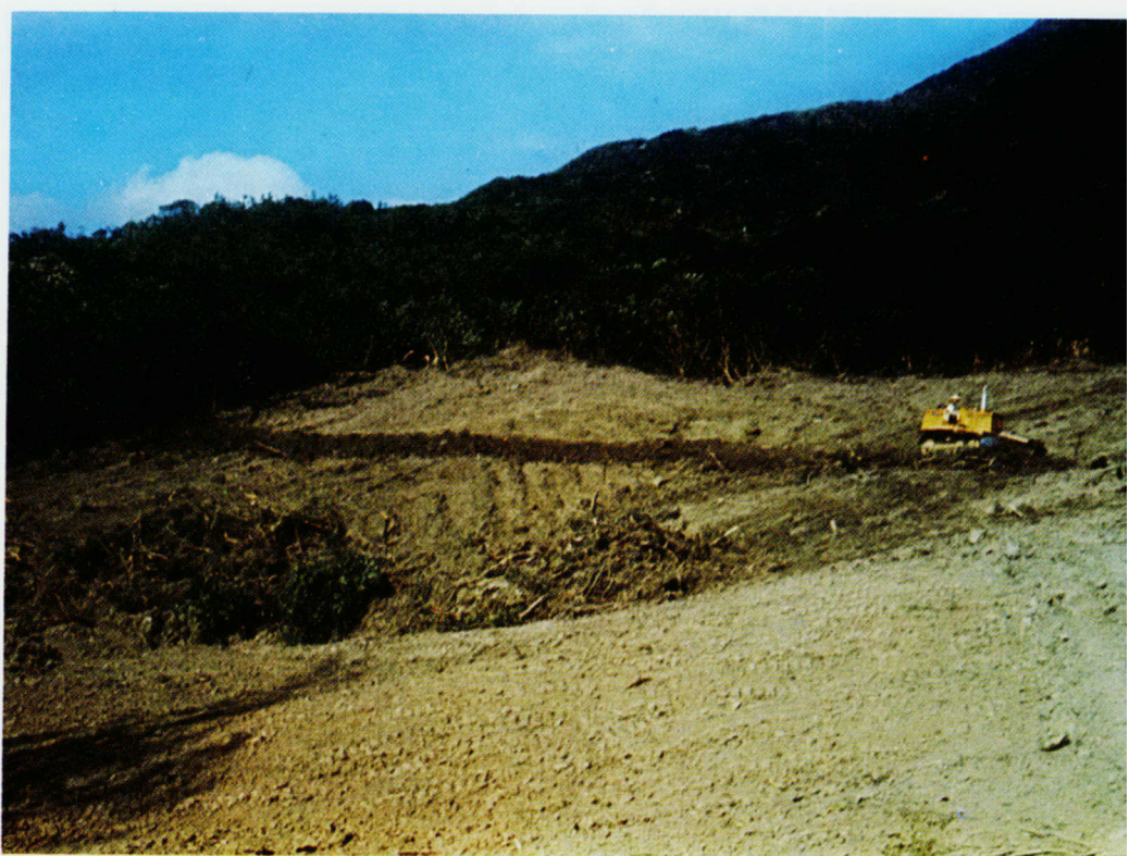
利用機械整理坡面及構築山邊溝。 Land levelling and hillside ditching by means of machines.
