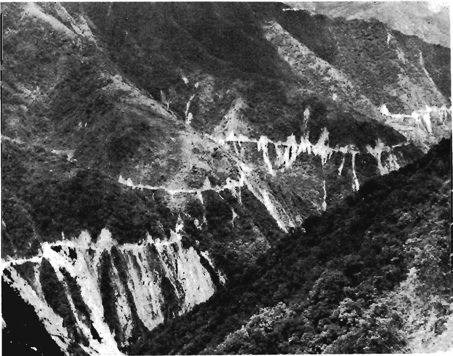
Plate 1-3. The Central Cross Island Highway created many landslides along its course in steep mountainous country.
