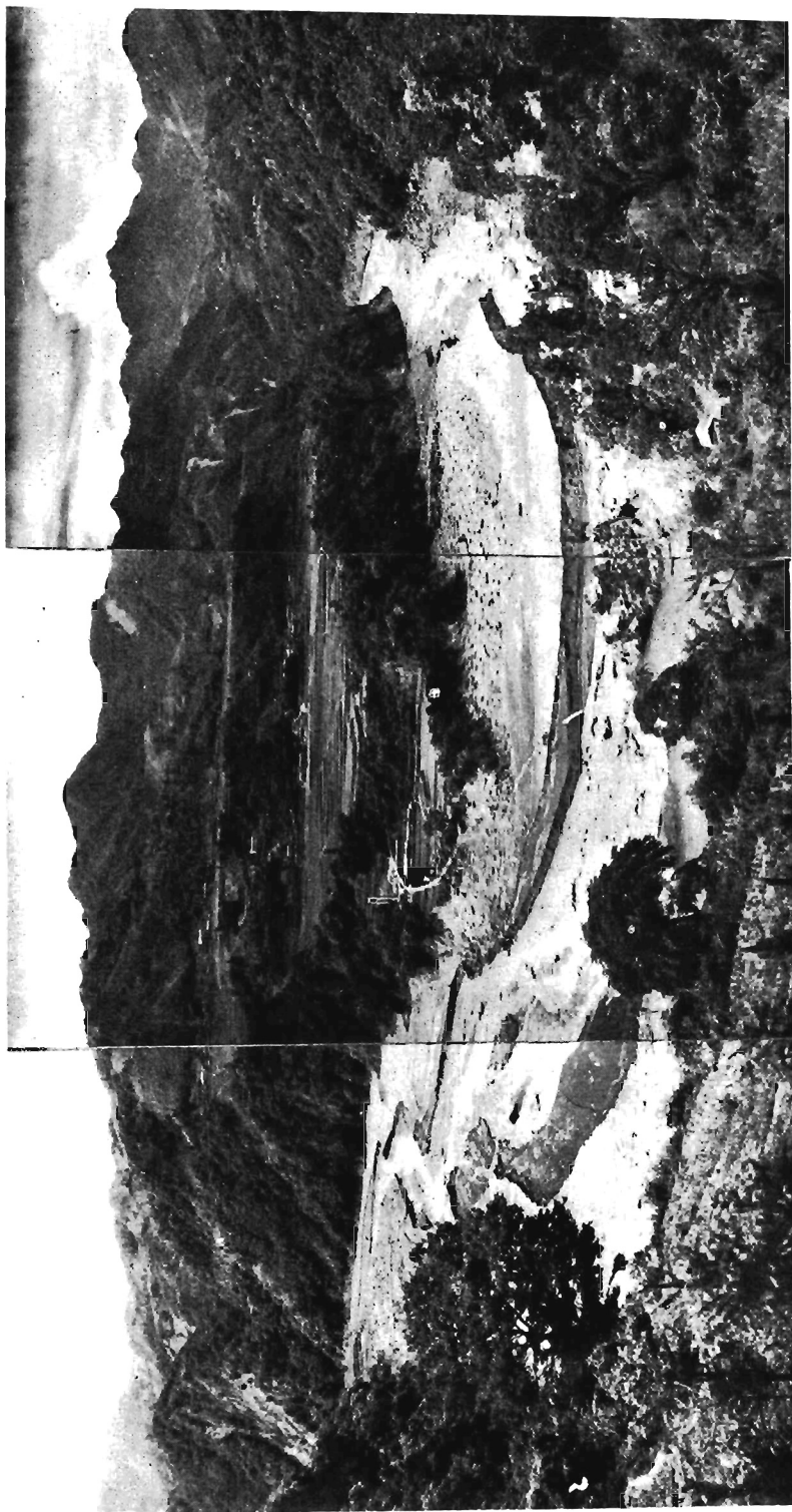
Plate 1-1. Heavy siltation occurred at the tail water of the newly completed Shihmen Reservoir. This was due to Typhoon Gloria which created hundreds of landslides in the watershed in September 1963.
